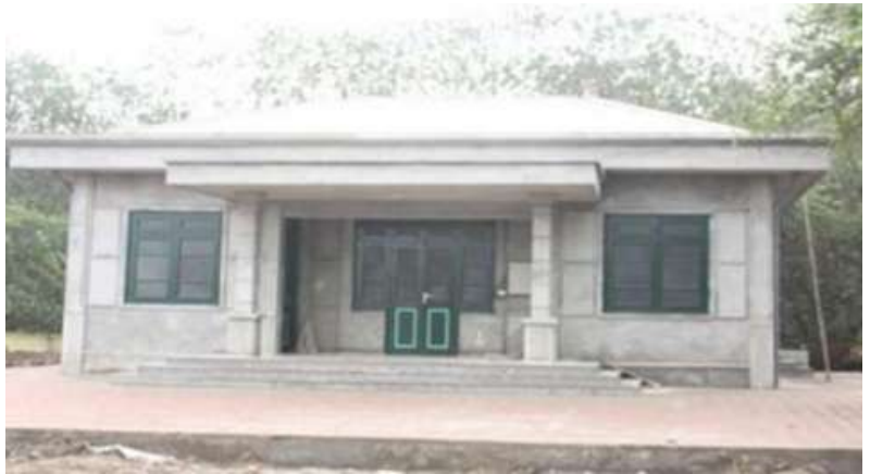
An execution compound in Vietnam
